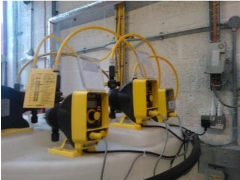
Diaphragm driven metering pumps have been the stalwart choice for dosing treatment chemicals ever since the Economic Boiler replaced the Lancashire and Cornish boilers.
