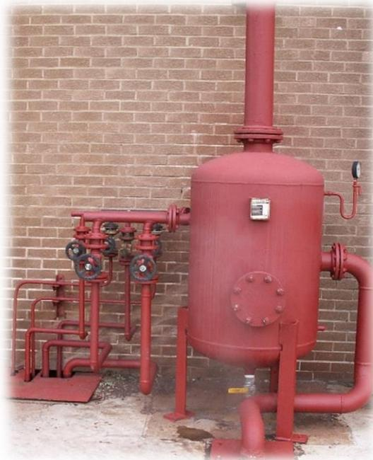
Apparently the UK system is better because it uses less cooling water. However, the initial cost for the vessel is higher and the installation is more expensive especially on multi-boiler sites where provision must be made to install the blowdown pipework beneath the boiler house floor in ducts or install a suspended floor to eliminate trip hazards. To assist cooling the blowdown vessel is frequently installed outside.
