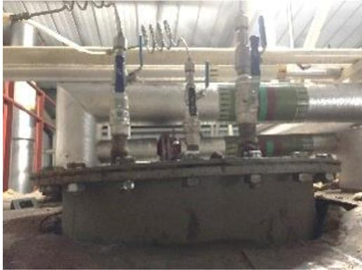
feeding chemicals direct to the feedtank with daily manual tests to ensure the parameters are met. Which are to ensure that there is no free oxygen in the boiler water, boiler pH is maintained between 10.5pH and 12.0pH and the dissolved salt level within the boiler is limited to between 3200ppm & 3500ppm.
